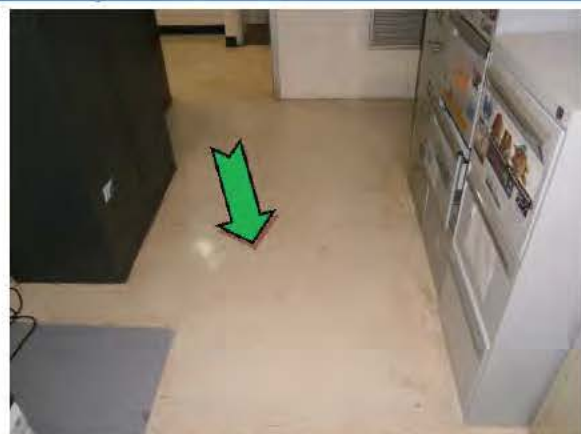
Photo 6. Ground level, throughout, floor coverings cream – non asbestos-containing vinyl floor tiles
