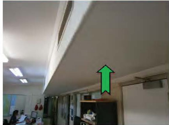
Photo 2. Ground level, throughout, air conditioning ductwork – non asbestos-containing fibre cement sheeting
