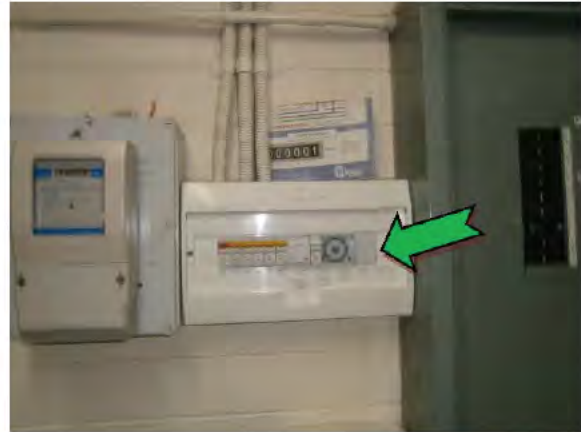
Photo 8. Ground level, printer room sub board, air conditioning unit – suspected non asbestos-containing bituminous backing board
