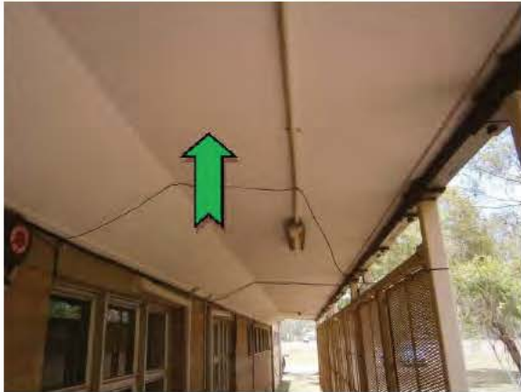
Photo 1. Ground level, throughout, eaves – non asbestos-containing fibre cement sheeting
