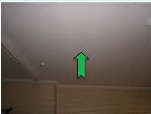
Photo 5. Ground level, throughout, ceiling – non asbestos-containing fibre cement sheeting
