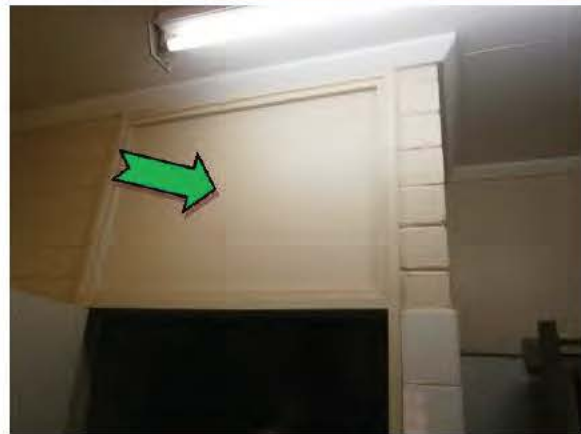
Photo 4. Ground level, men's toilet, infill panels high level – non asbestos-containing fibre cement sheeting
